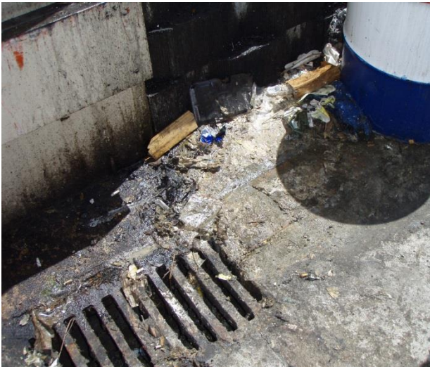
Make sure food waste, grease and fats do not go down drains
