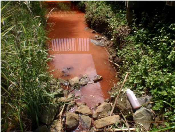
Run-off from waterblasting a terracotta roof which went into a stream, causing pollution
